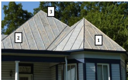
Historic standing-seam metal roof
