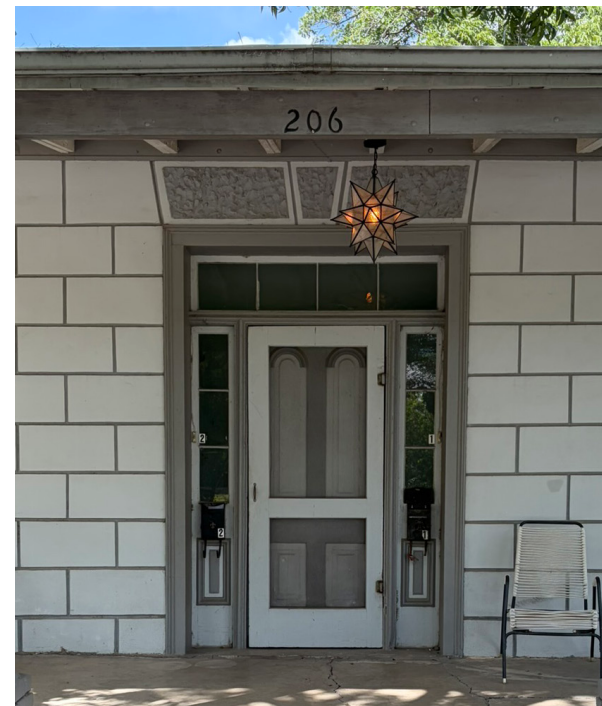
Existing Front Door
