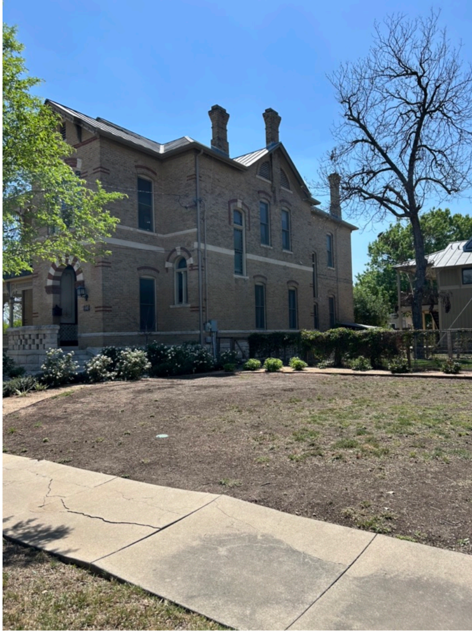
Side Facade - North Elevation
