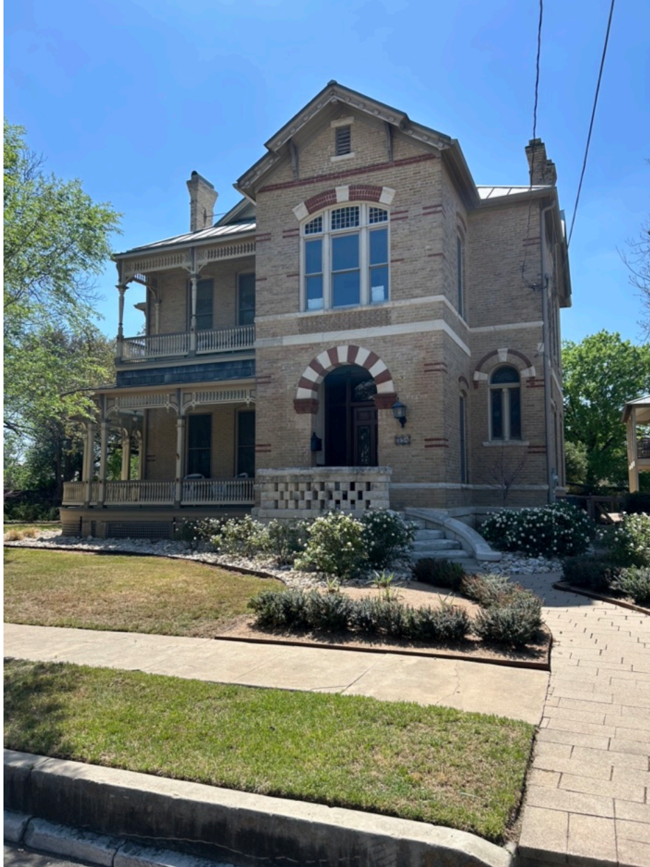
Front Facade Facing Adams Street - East Elevation
