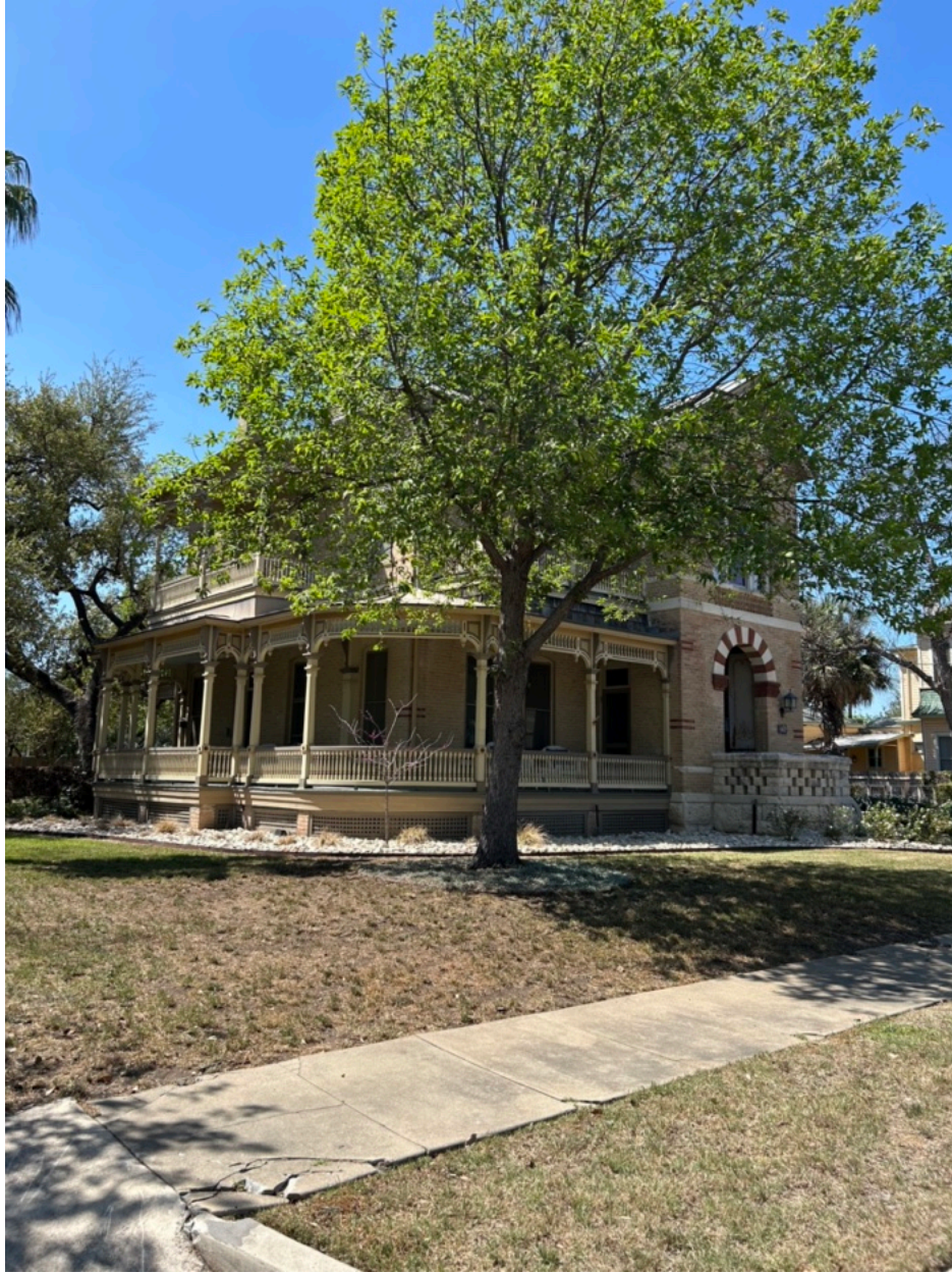
Side Facade - South Elevation
