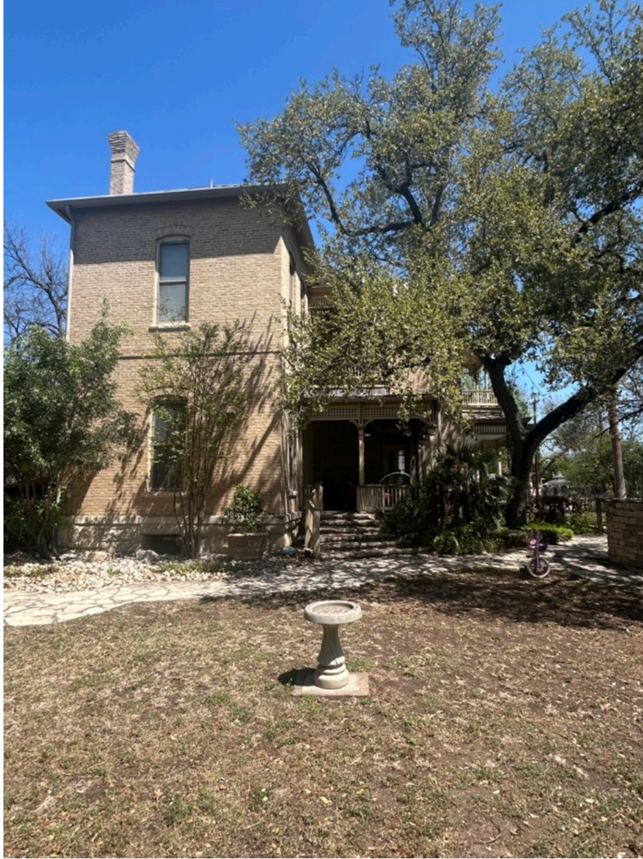
Rear Facade - West Elevation
