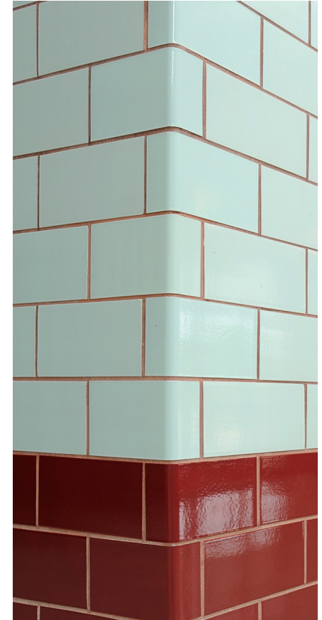
GLAZED MASONRY INTERIOR
