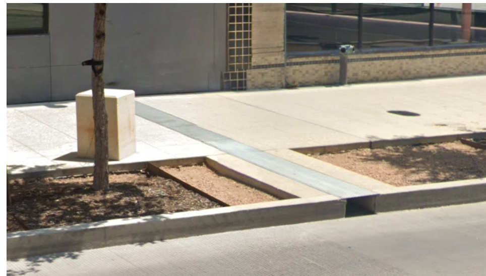
③ Zona Cultural metal roof drain (thorough planting area) Also observed square concrete curb
