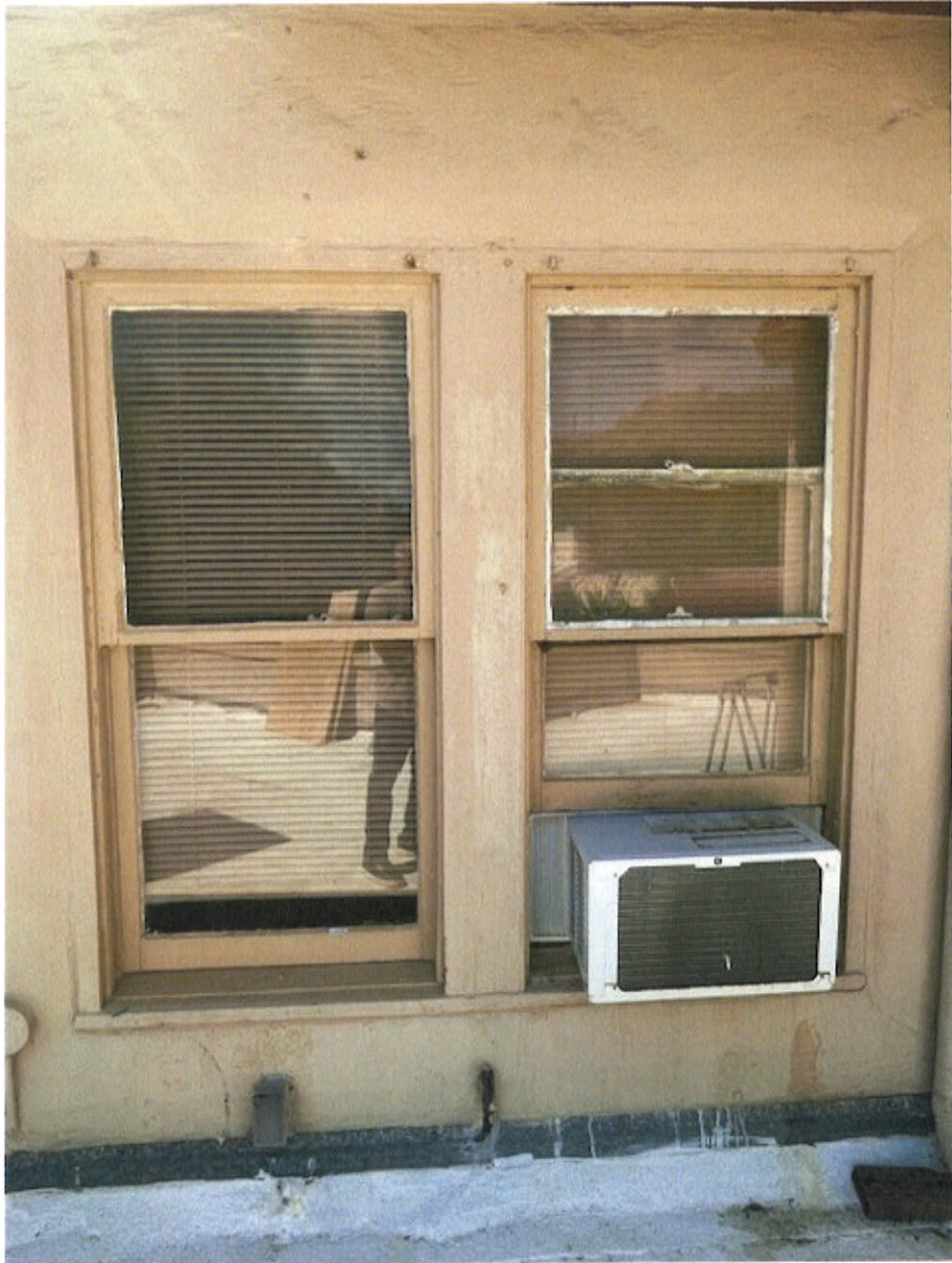
2nd Story Primary Bedroom East
