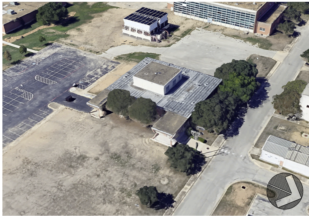
AERIAL VIEW LOOKING WEST
