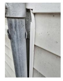
Location: Near Kitchen Door Notes: Vinyl siding is pulled up, exposed felt barrier behind. Improper termination of felt has led to potential moisture intrusion
