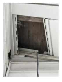
Location: **Exterior of Guest Room (soffit)** Notes: -Gap in siding has exposed wooden eaves -Pest intrusion concern
