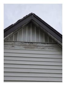
Location: Front face of house Notes: -Storm damage has ripped top vinyl panel & moulding off. -Exposure to outside conditions has deteriorated wood -Original wood lap siding exposed.
