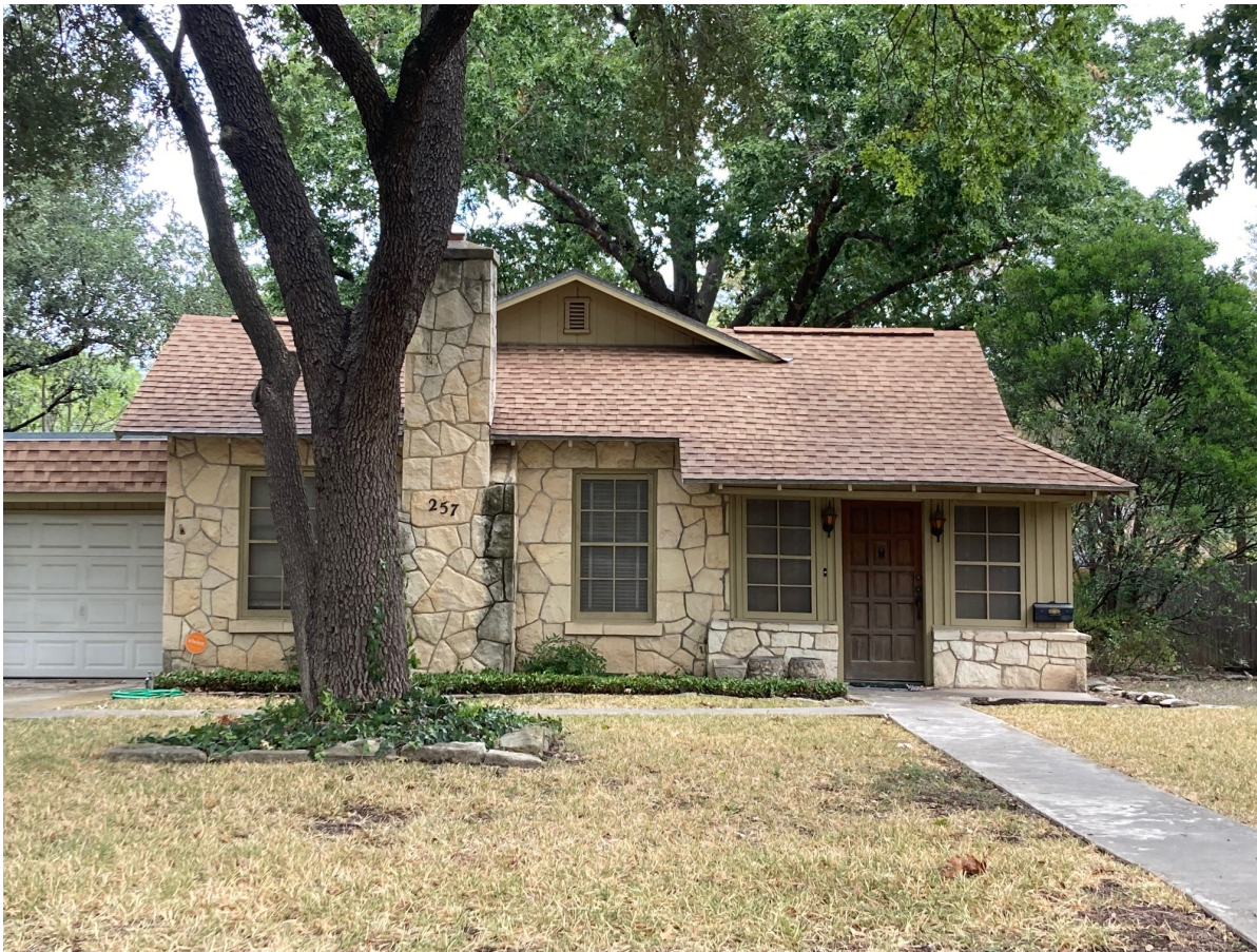
Fully converted front porch.
