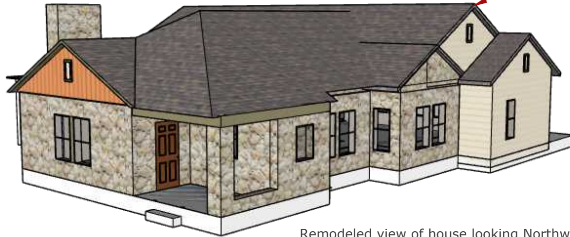
Remodeled view of house looking Northwest.
