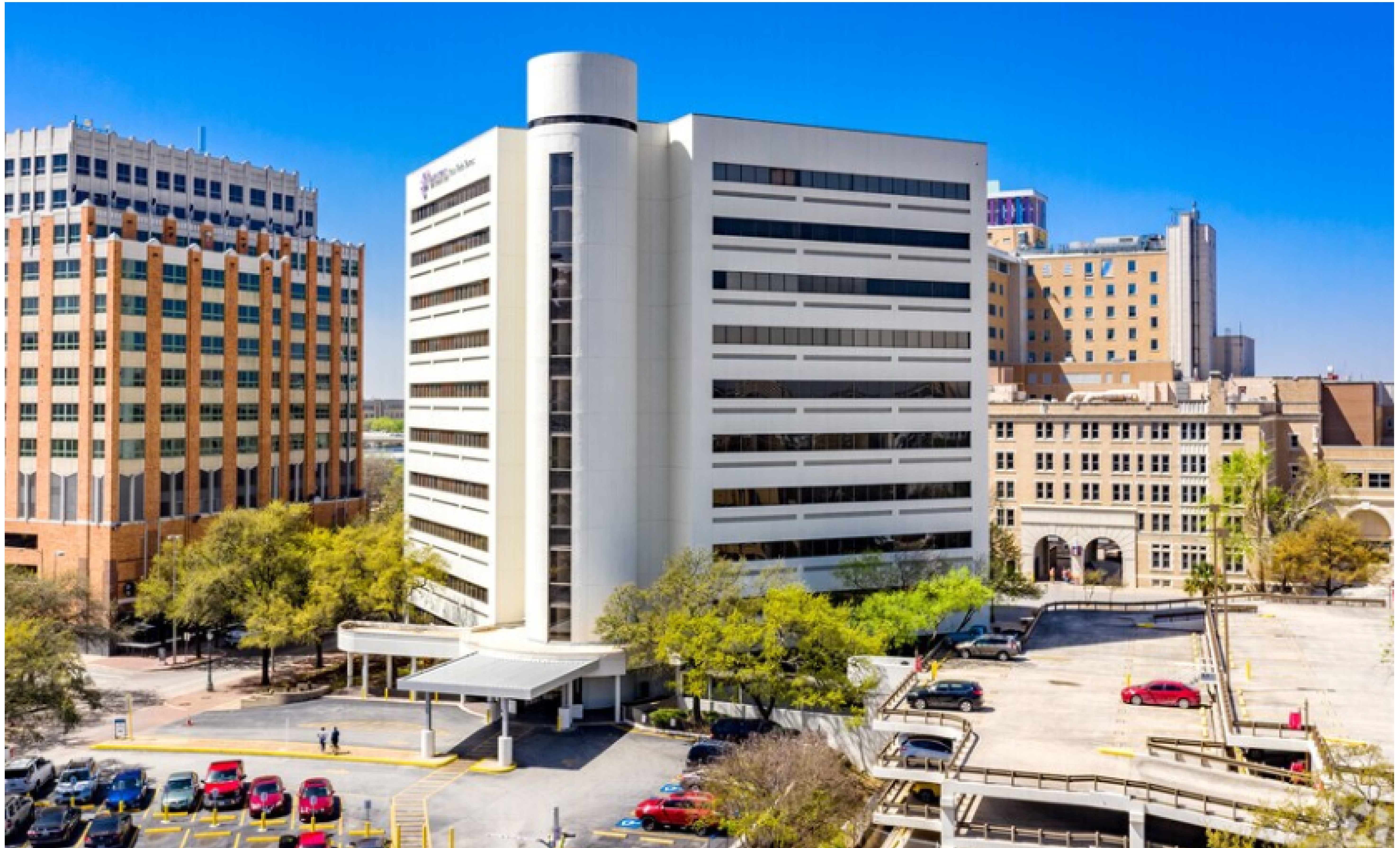
VIEW FROM SAN PEDRO CREEK
