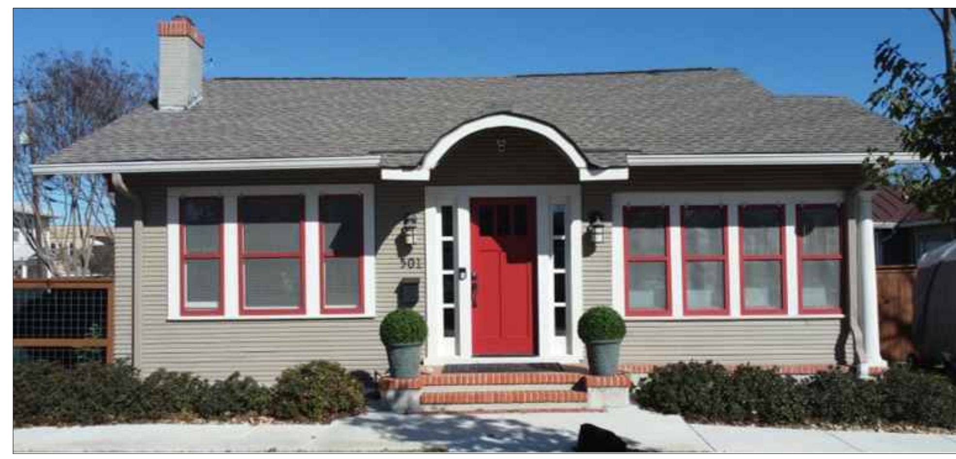
Existing Porch Photo Reference
