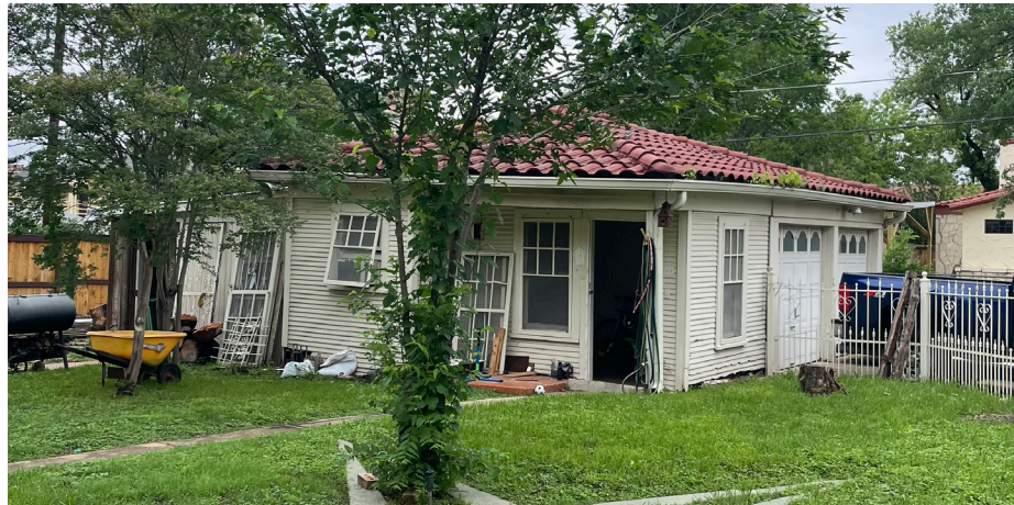
1. SOUTH FACADE OF EXISTING ADU
