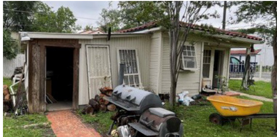
2. SOUTH FACADE OF EXISTING ADU
