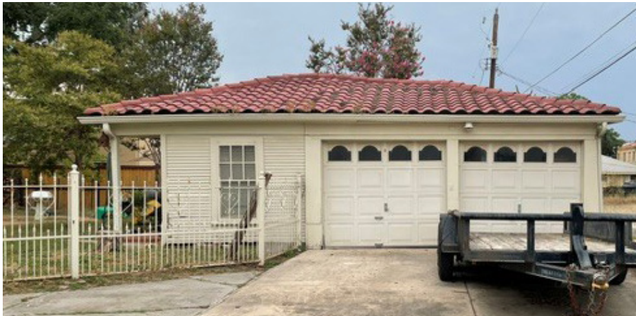
3. EAST FACADE OF EXISTING ADU
