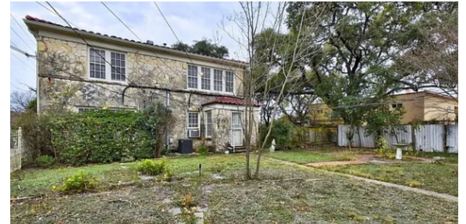
3. NORTH FACADE OF PRIMARY STRUCTURE
