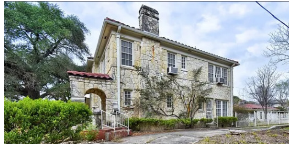
2. EAST FACADE OF PRIMARY STRUCTURE
