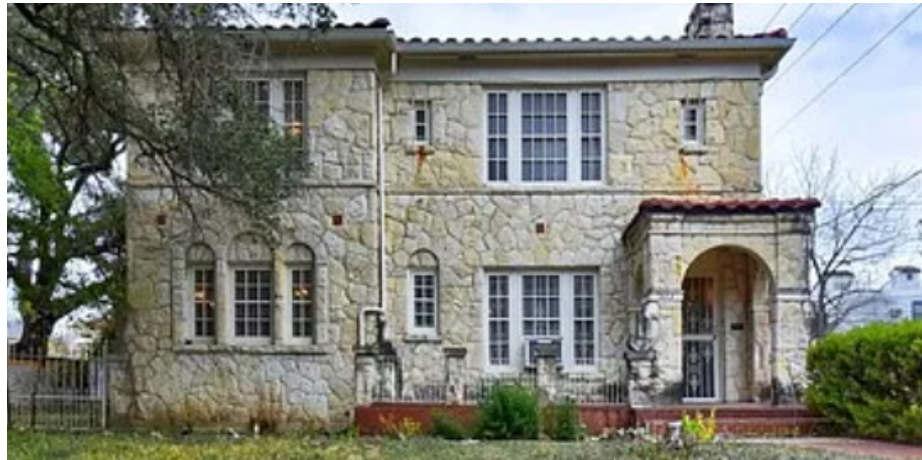
1. SOUTH FACADE OF PRIMARY STRUCTURE
