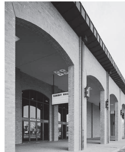
Columnades of standard clay brick (pilasters and walls)
