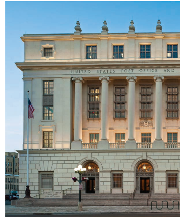
Hipolito Garcia Federal Building (Limestone cladding)
