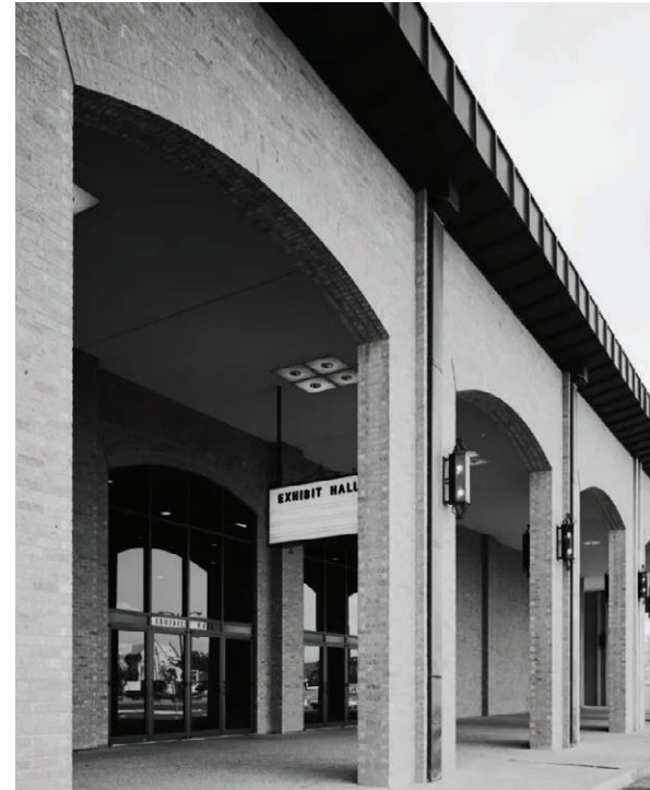
'68 Convention Center (Covered porticos)
