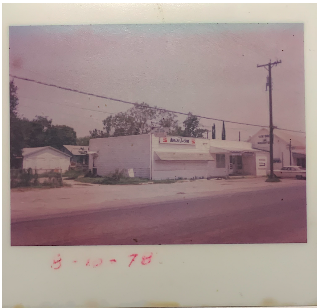
View of 920 and 922 Clark Ave from the Northwest. Photo taken from Clark Ave. August 10, 1978. Source: Michael Quiroz family/research archive.
