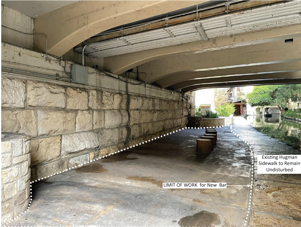
Existing Sidewalk (South side of Riverwalk) looking West
