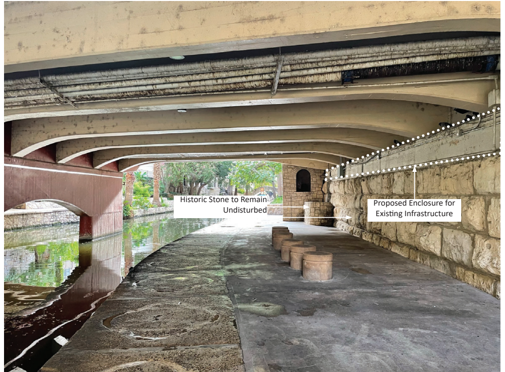
Existing Sidewalk (South side of Riverwalk) looking East
