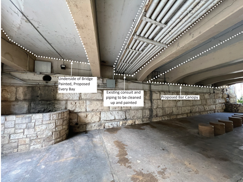
Existing Elevation, Looking South
