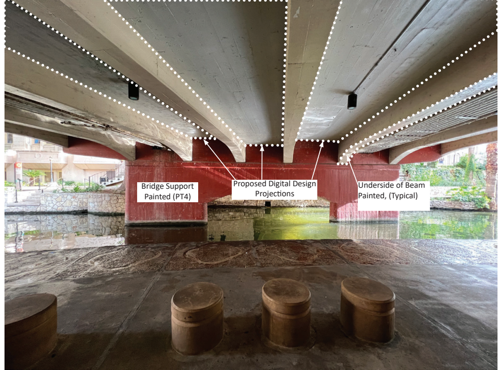
Existing Elevation, Looking North
