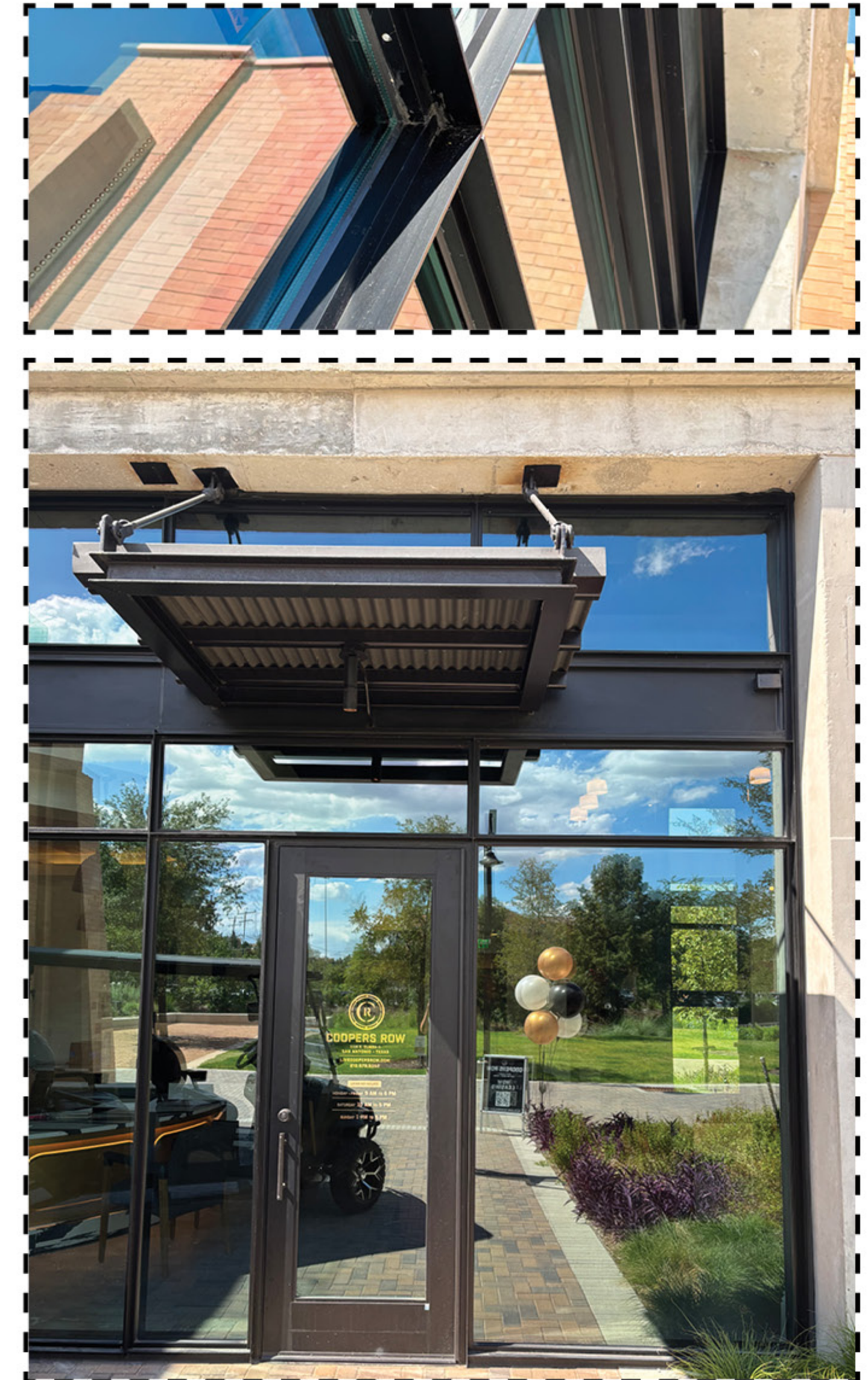
ALUMINUM STOREFRONT WITH UPGRADED PRESSURE PLATE - EFCO 5600 - PROFILE 6337 COLOR: CUSTOM BAKED
