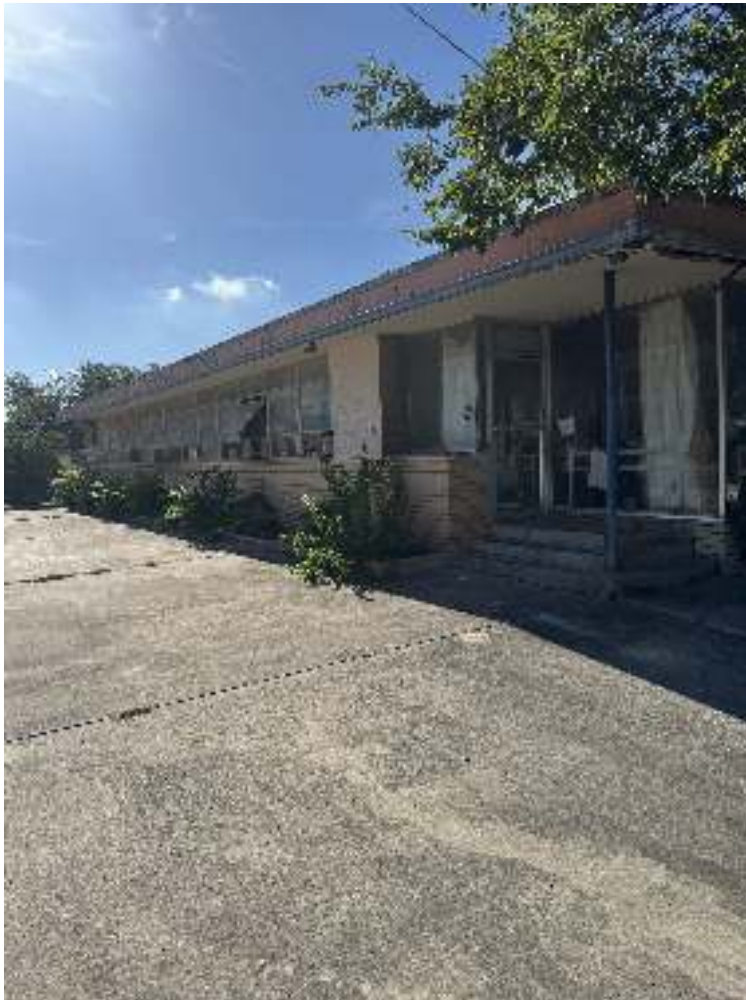
Closer oblique view of the entry bay at the west end of the primary (north) facade, showing the cantilevered canopy, plate-glass storefront, reception doors, and the brick end-pier with "538" address numerals. Roman brick bulkhead and steel-sash transom windows are visible. Taken April 2026.
