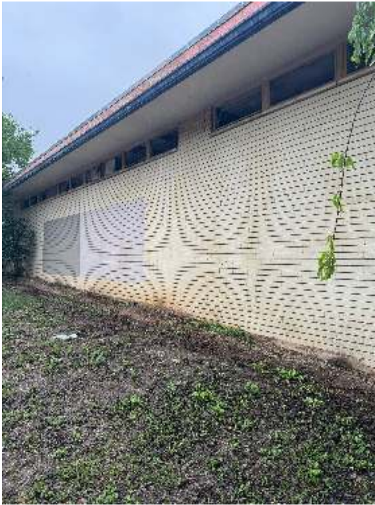
View looking east from N. Flores Street. The full-length clerestory ribbon of steel-sash windows runs below the eave across the entire west elevation, providing daylight to the open work room. Buff Roman brick wall with minimal openings at grade. Taken April 2026.
