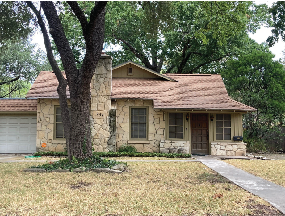
Fully converted front porch.
