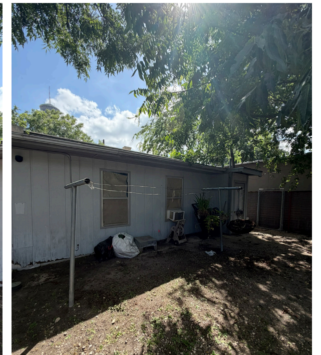
Existing Rear Addition
