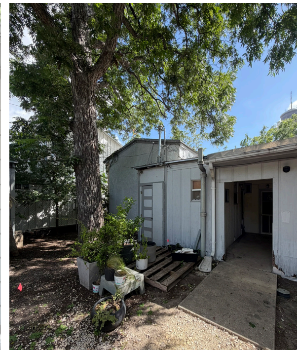
Existing Rear Addition
