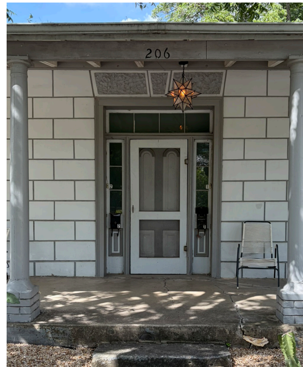
Lavaca St. Entry
