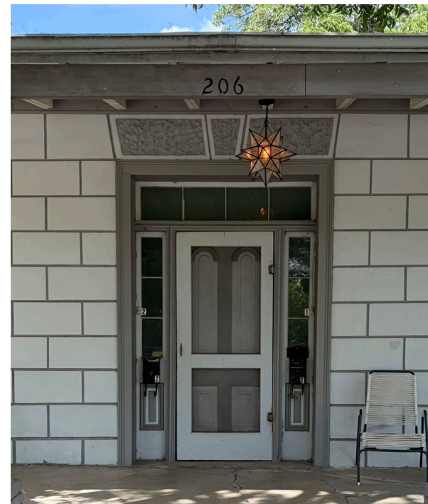
Existing Front Door
