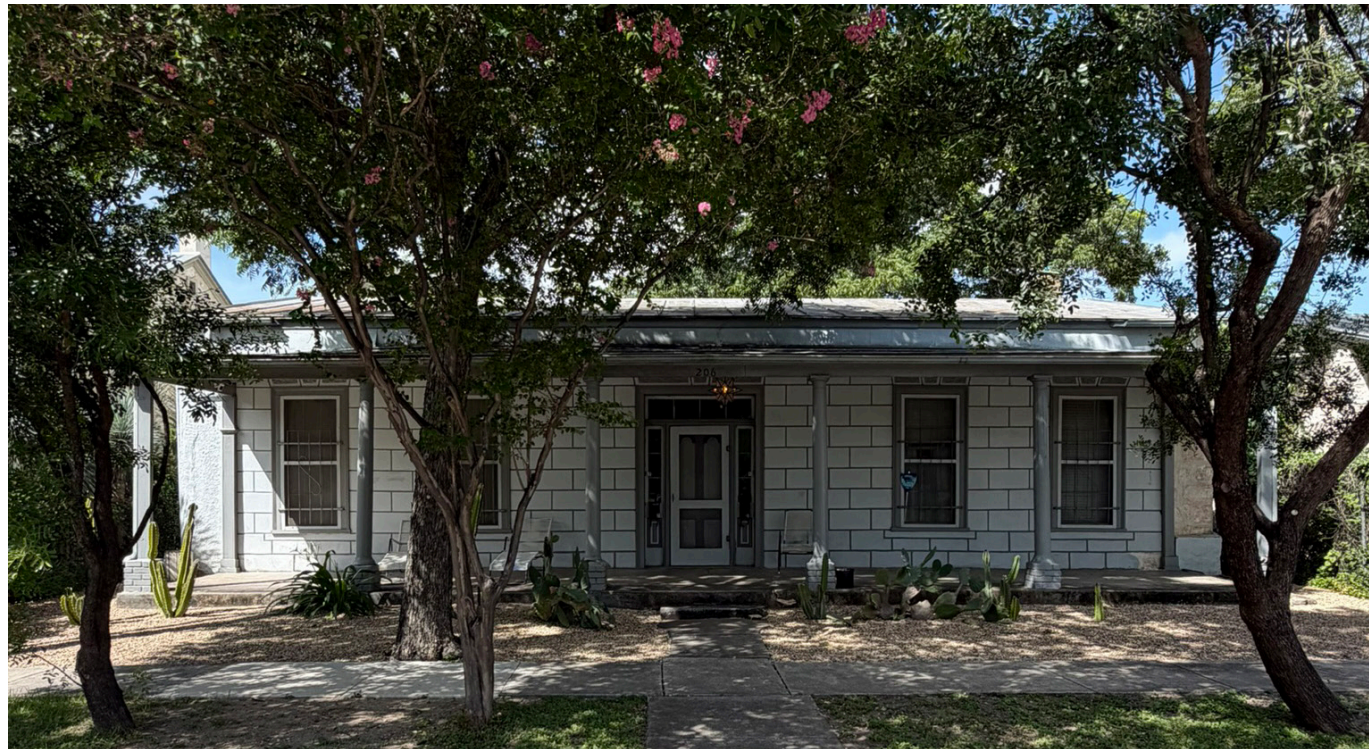
Front Elevation from Lavaca Street
