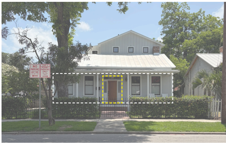
126 Barrera 21'-0" wide facade 5'-0" wide door + sidelites 16.7%
