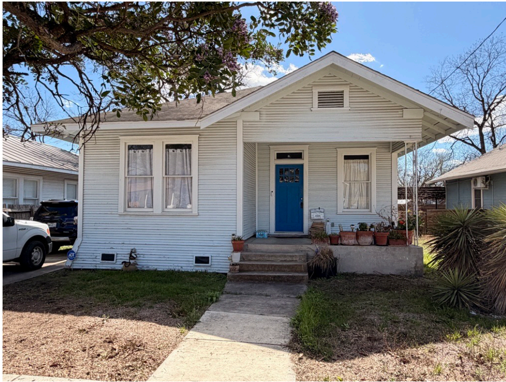
EXISTING PRIMARY STRUCTURE
