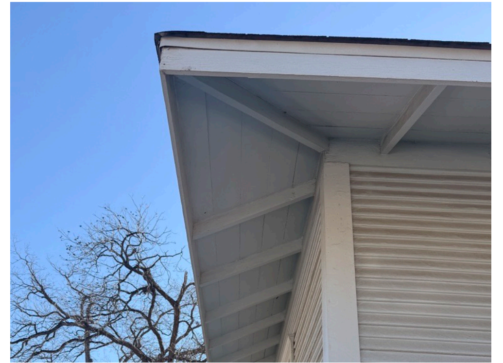
EXISTING PRIMARY STRUCTURE
