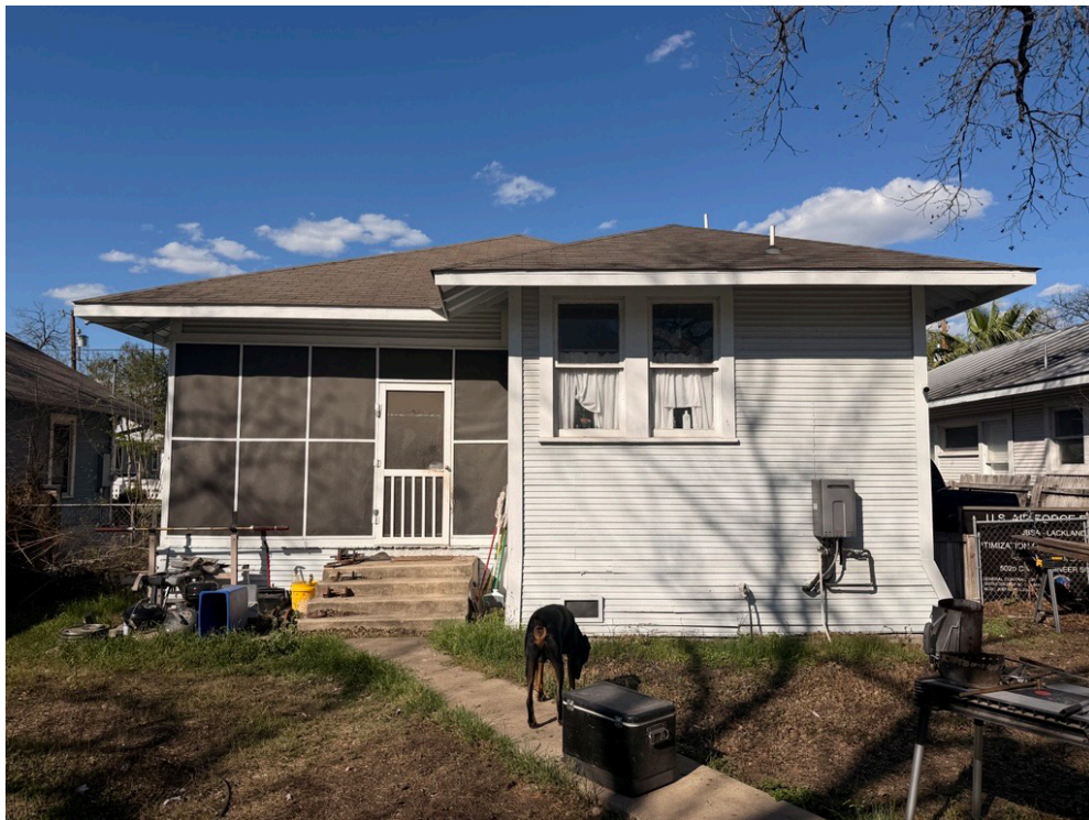
EXISTING PRIMARY STRUCTURE
