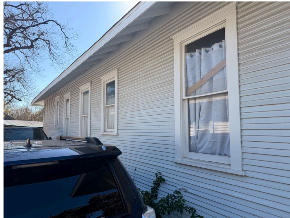
EXISTING PRIMARY STRUCTURE
