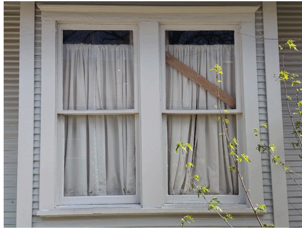
EXISTING PRIMARY STRUCTURE
