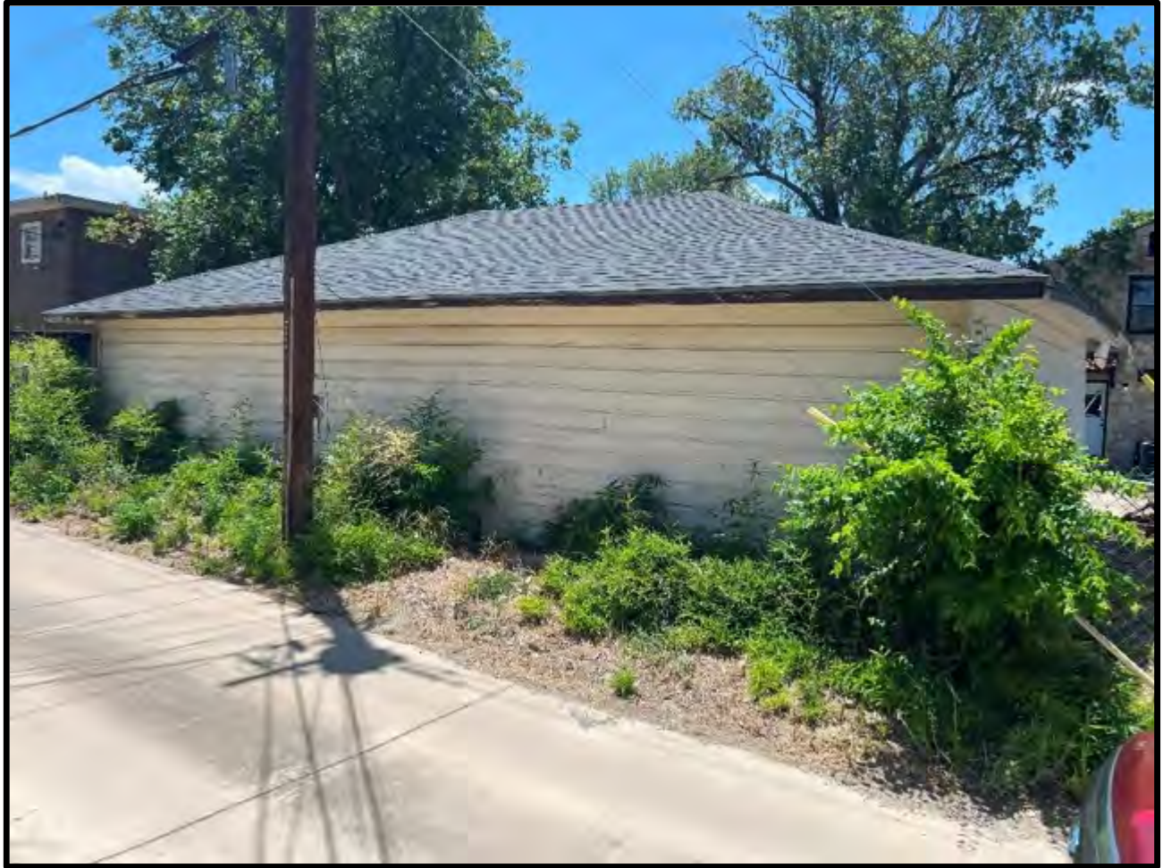
View of the rear (north) elevation of the detached garage building.
