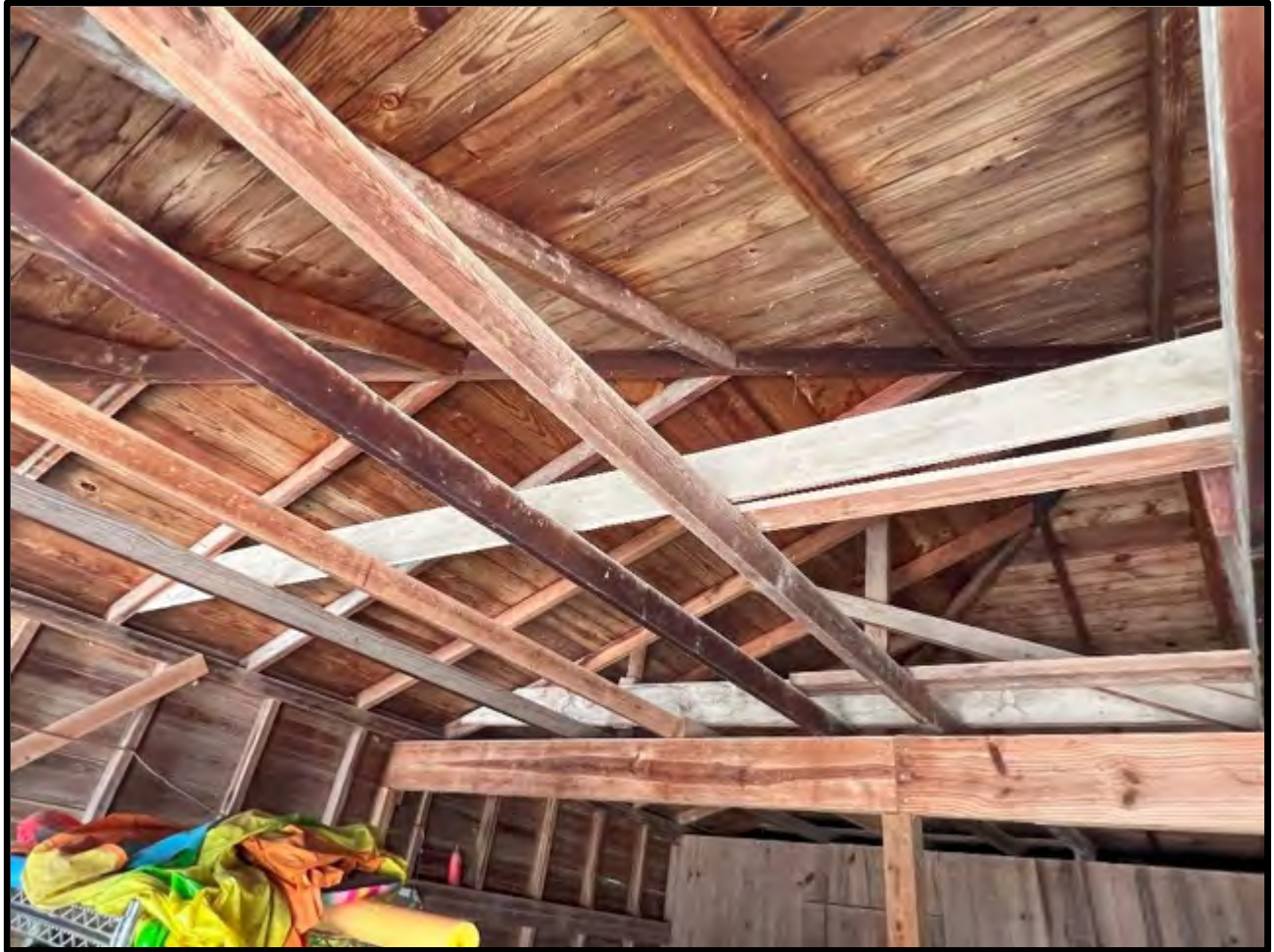
Overview of the interior framing of the detached garage building.
