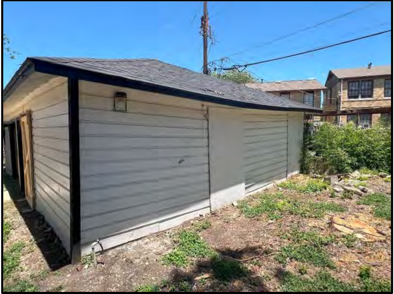
View of the right side (east) elevation of the detached garage building.
