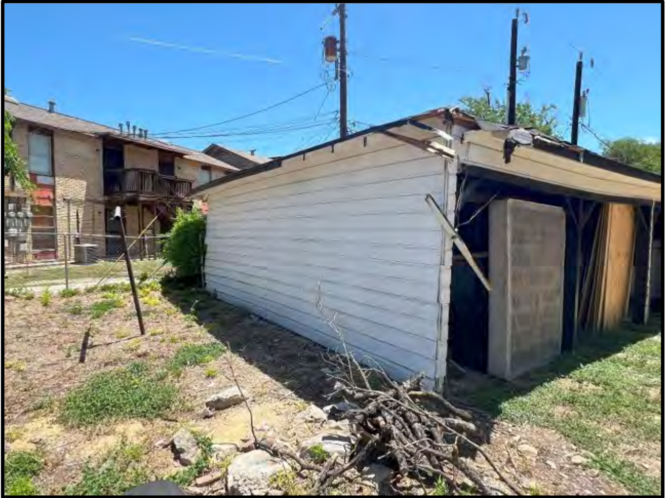
View of the left side (west) of the detached garage building.
