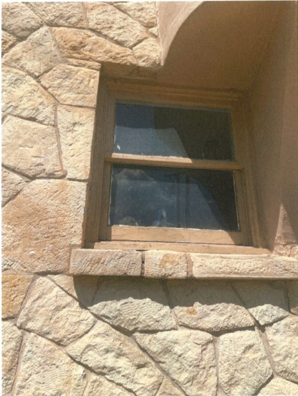
1st Floor Kitchen Sink
