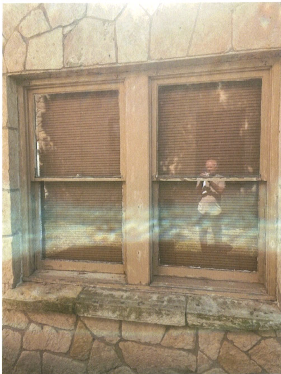
1st Floor Office East
