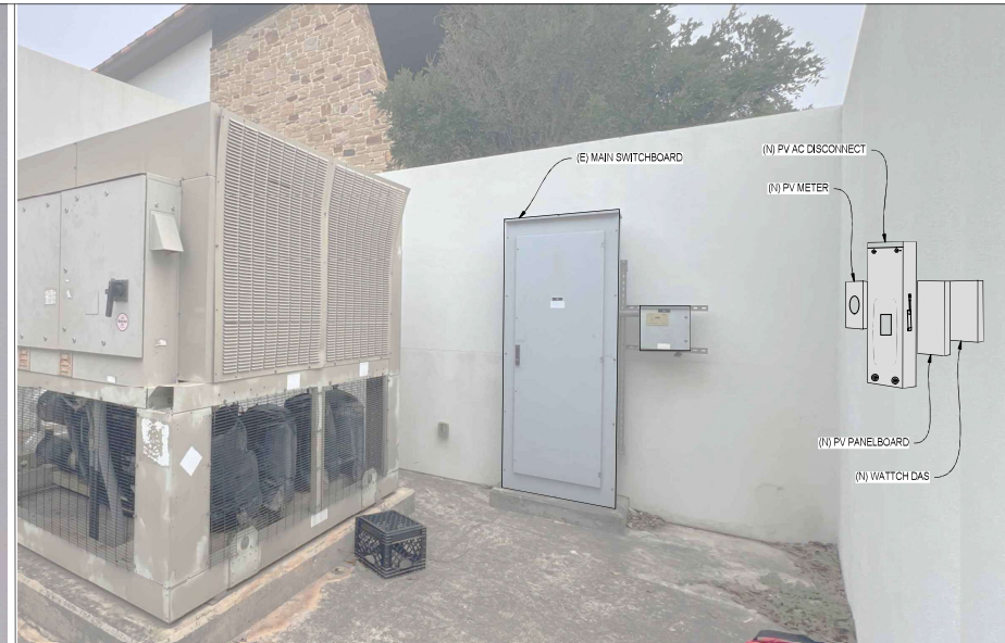
C EQUIPMENT ELEVATION-3 (EXTERIOR)
