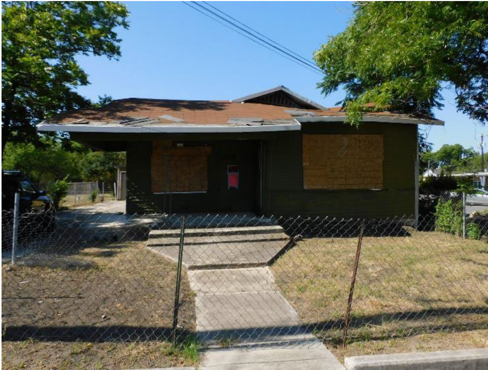
Photo 1, North elevation, overall (front).
