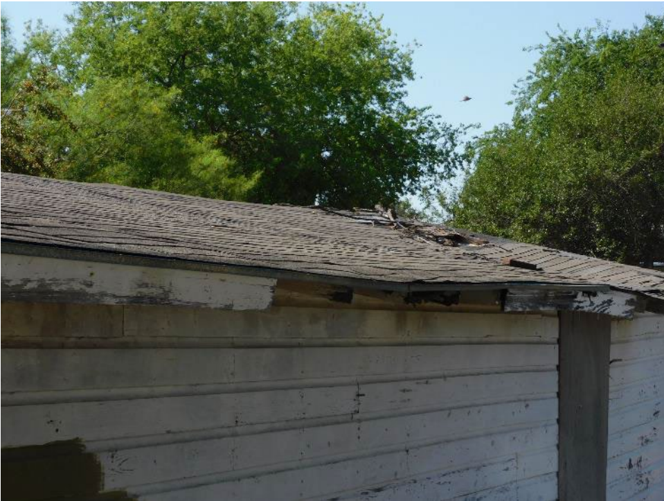
Photo 13, Exterior, garage roof.
