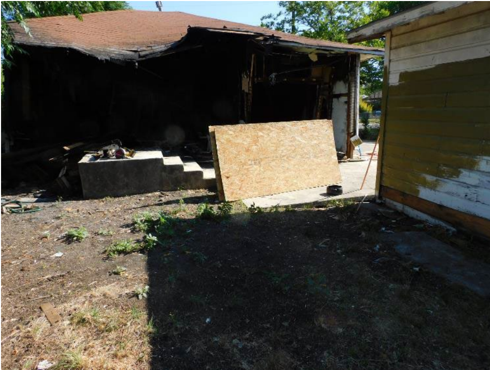
Photos 3, South (rear) elevation.
