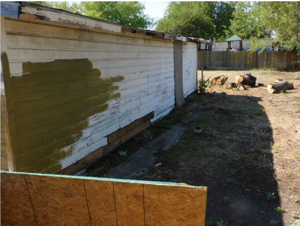
Photo 14, Exterior, garage cladding.
