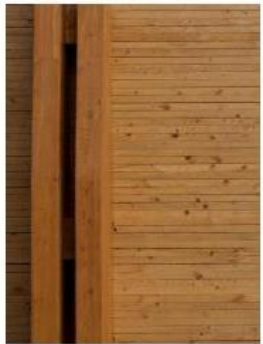
GLULAM & CLT DECK
