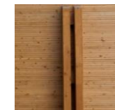
4. Glulam + CLT deck
