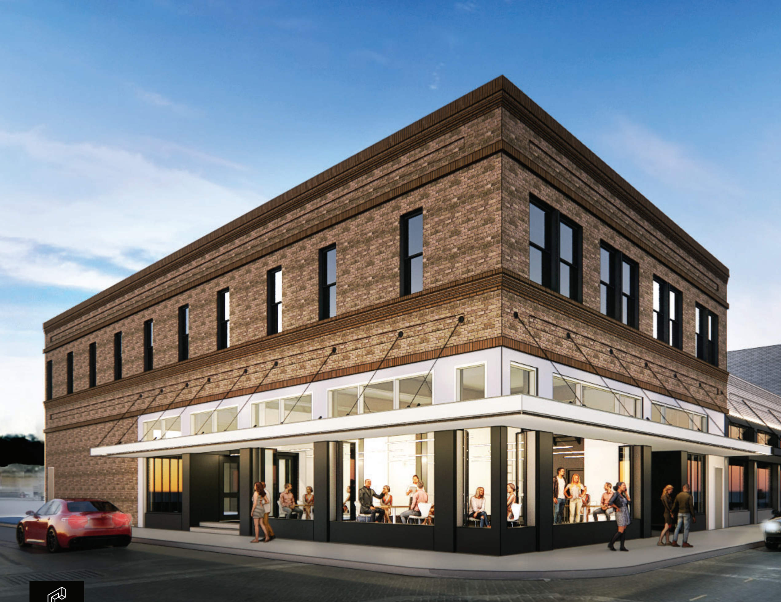
LINEAR LED IN SOFFIT
