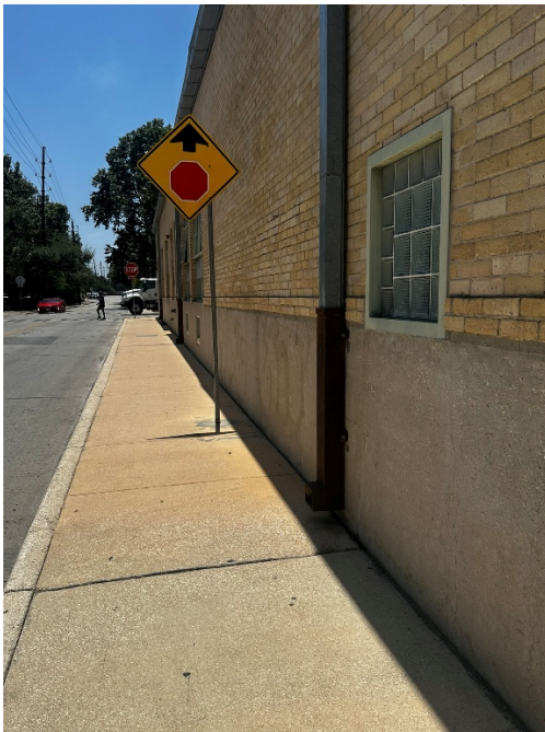
Figure 5. Sidewalk provides less than 6 feet of width for pedestrian travel, not including existing signage. Current configuration also does not provide any shade.
