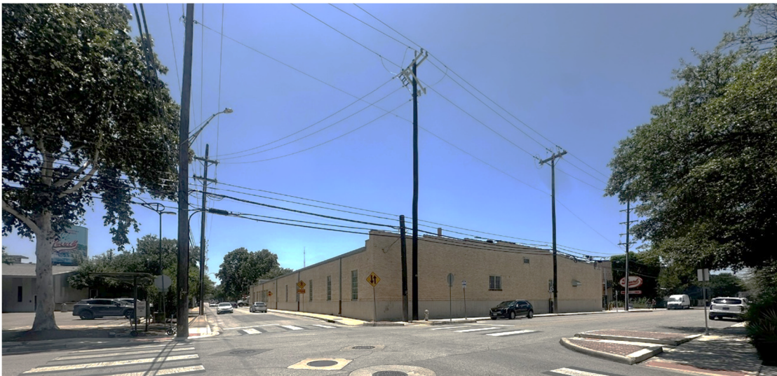
Figure 1. View of the Garage Building from the northeast corner shows elevated slab and lack of permeability and connection to passersby. Configuration of the building close to curb does not allow for pedestrian connections to building (stairs and ramps are not physically possible).
