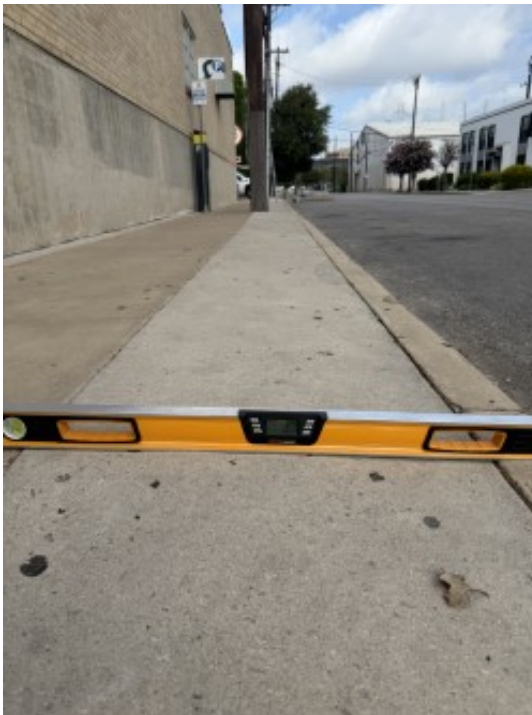
Figure 3. Cross slope of 5% on additional sidewalk is not ADA compliant.
