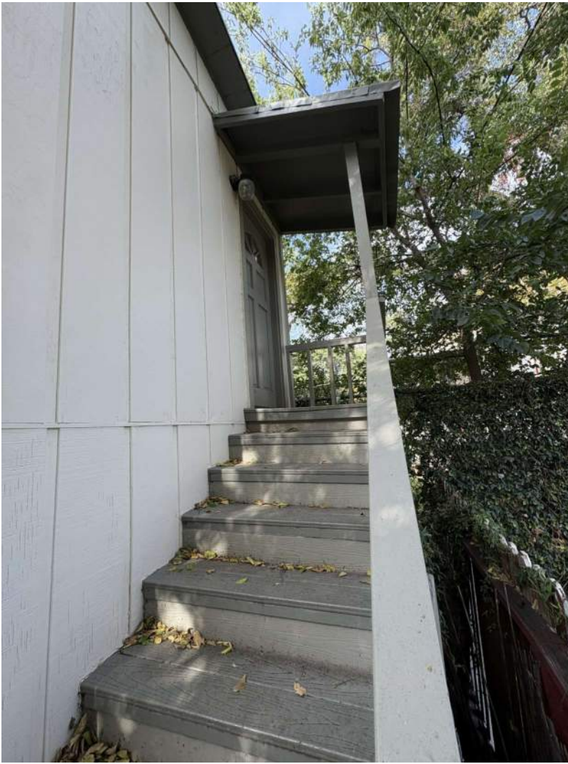
NORTH FACADE AND STAIR OF CARRIAGE HOUSE.
