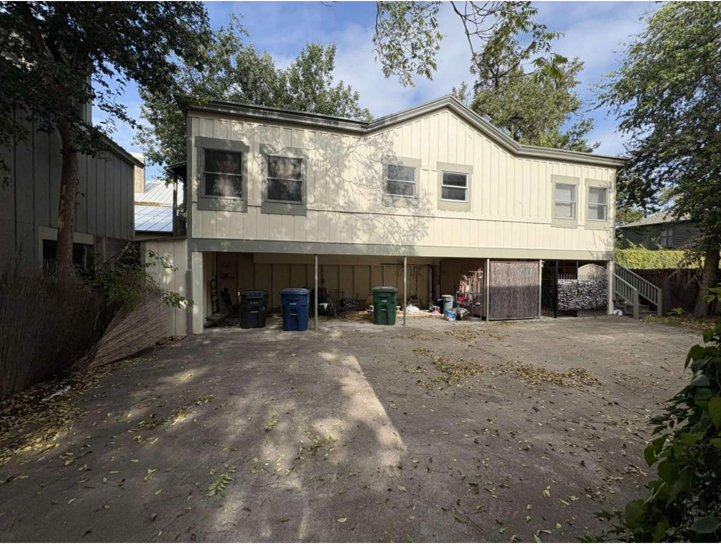
EAST FACADE OF CARRIAGE HOUSE.
