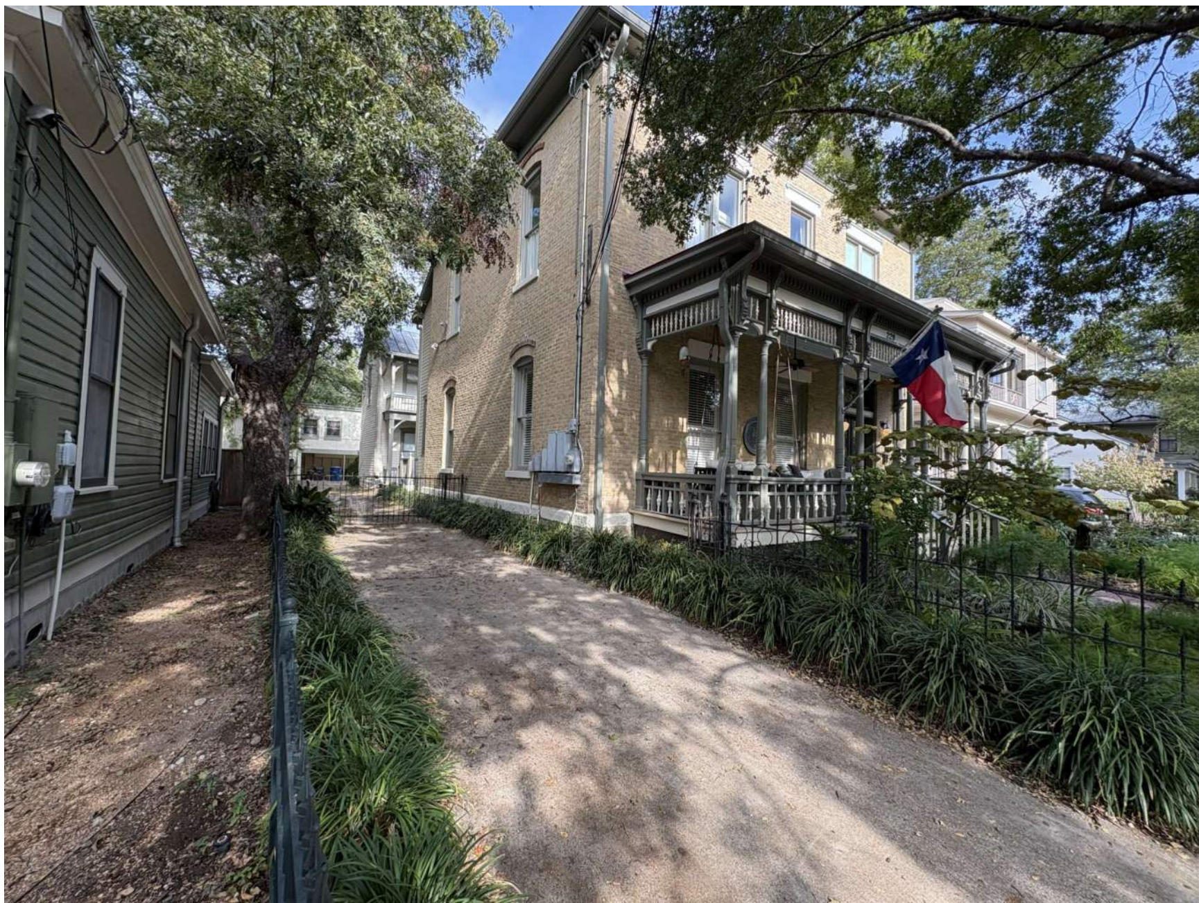
SOUTH FACADE OF MAIN HOUSE FROM DRIVEWAY ENTRANCE.
