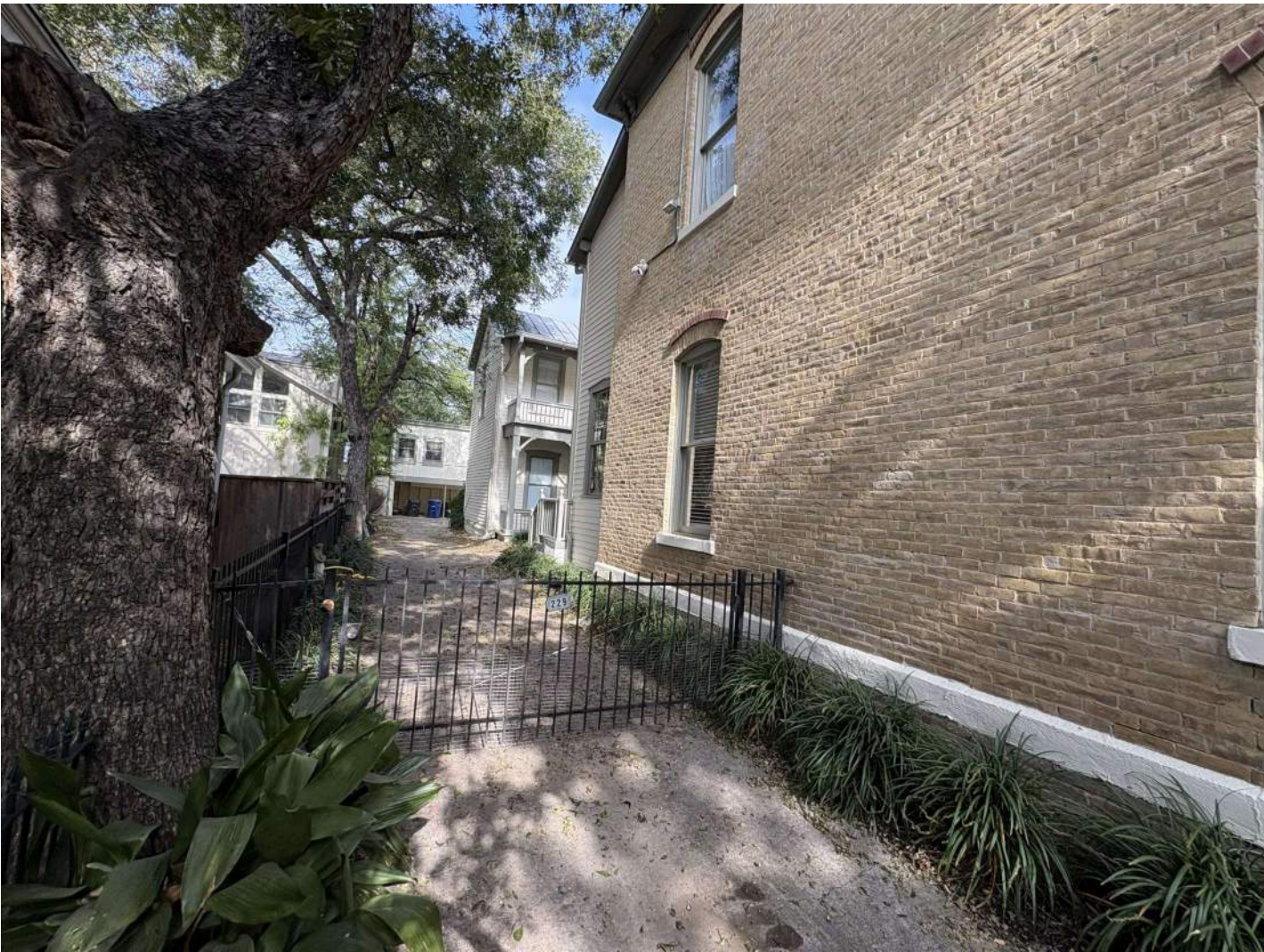
SOUTH FACADE OF MAIN HOUSE - VIEW OF COURTYARD & CARRIAGE HOUSE BEYOND.
