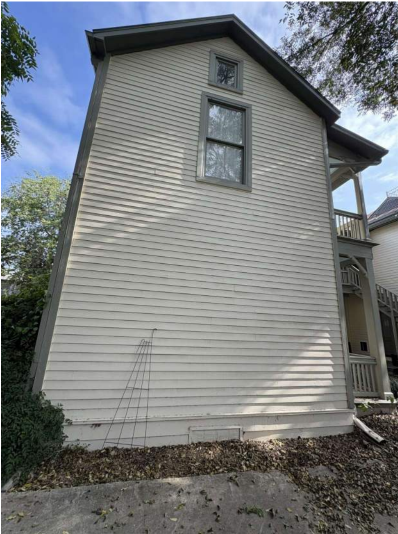
SOUTH FACADE OF 1990s ADDITION.
