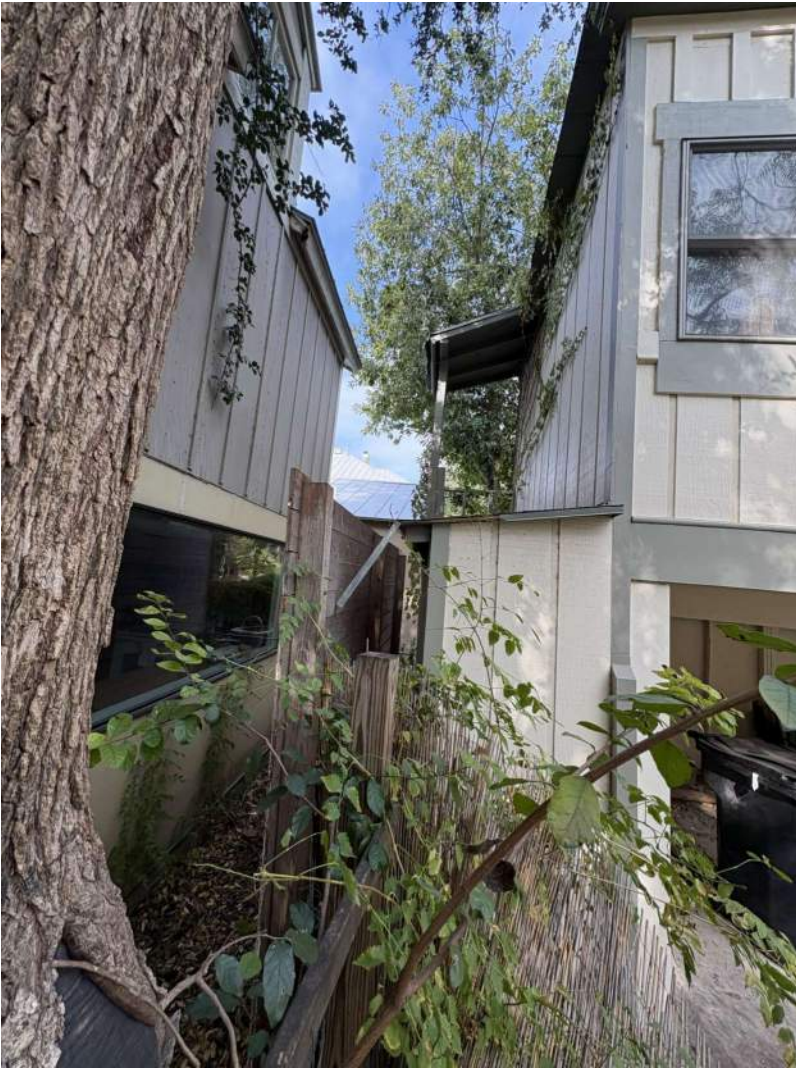
SOUTH SIDE YARD NEXT TO CARRIAGE HOUSE.
