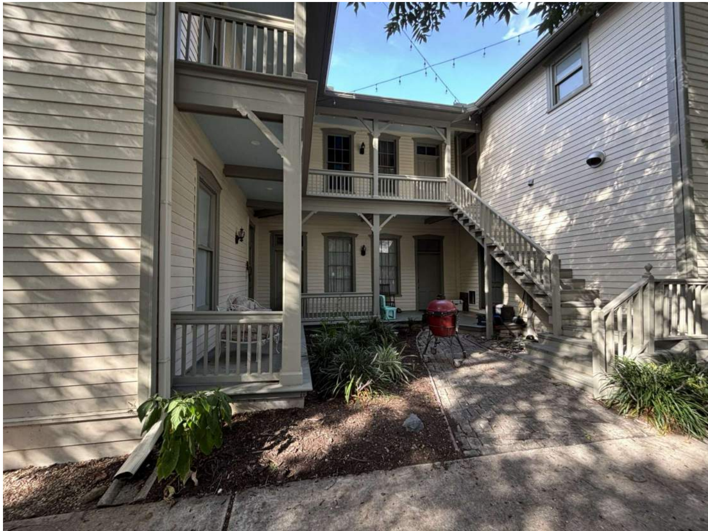
VIEW INTO EXISTING COURTYARD.
