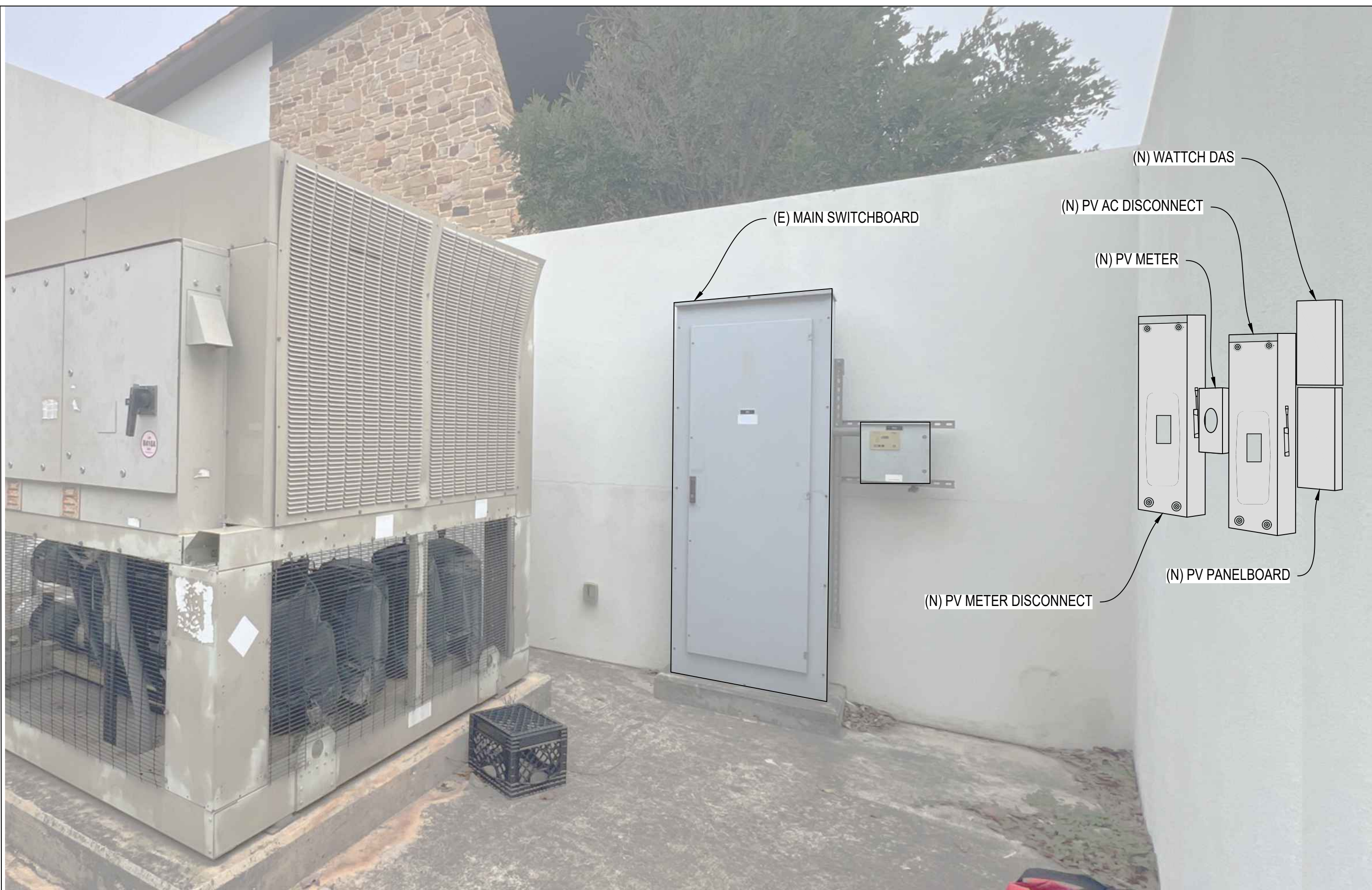
C EQUIPMENT ELEVATION-3 (EXTERIOR)
