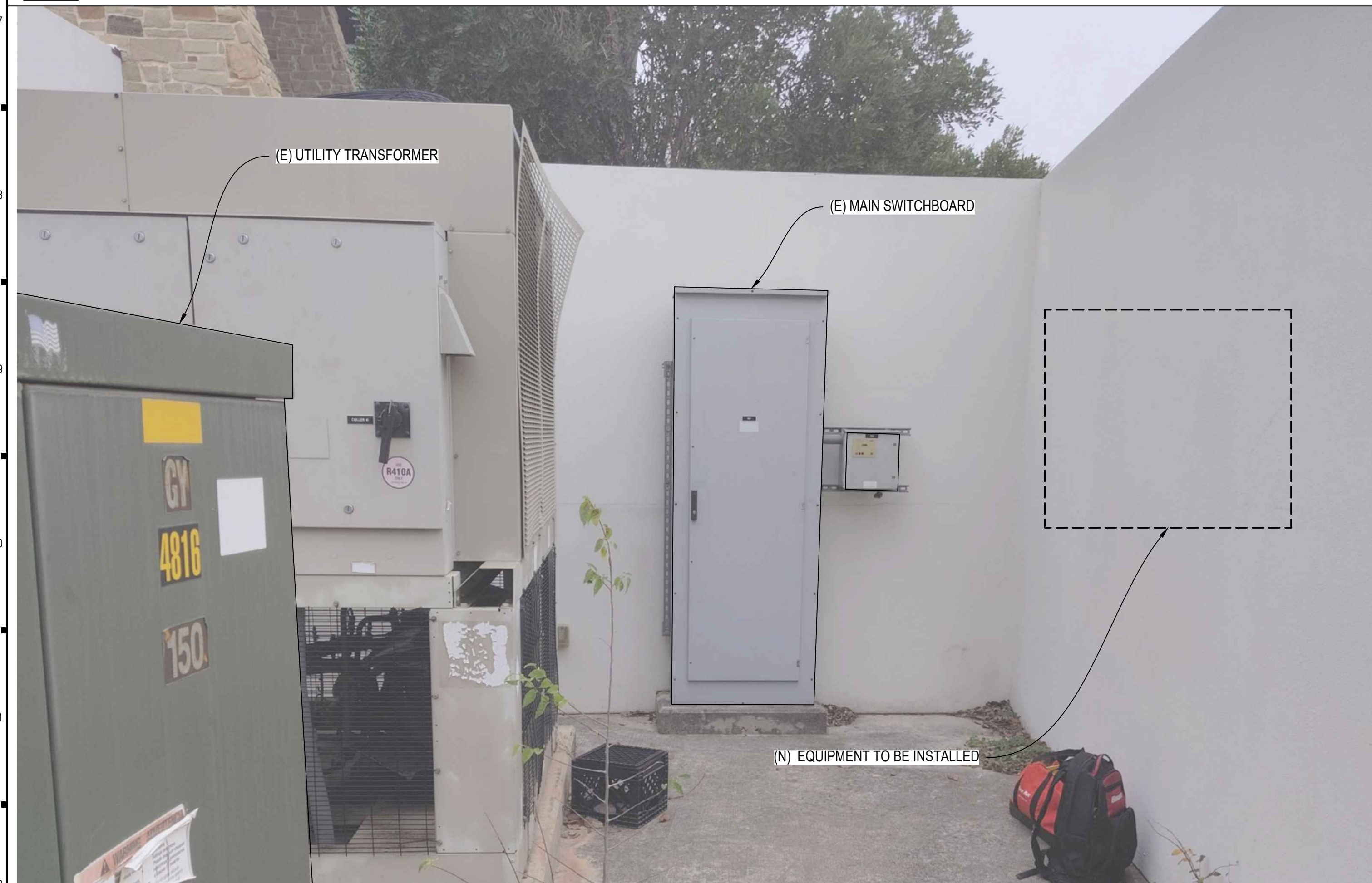
B EQUIPMENT ELEVATION-2 (EXTERIOR)
