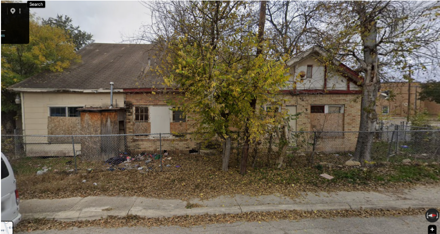
EAST FACING SIDE (HANDLEY ST)
