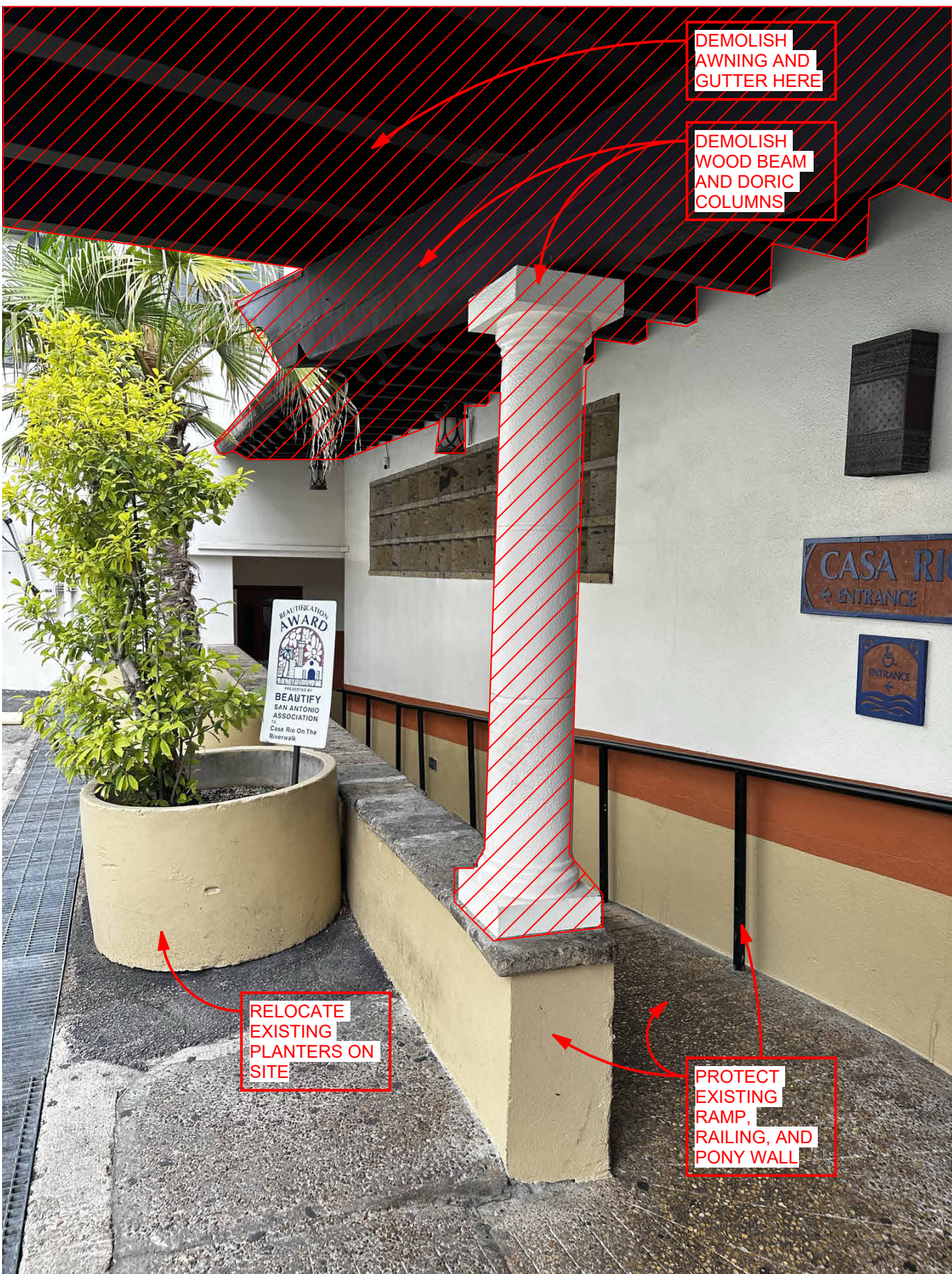
5. VIEW OF EXISTING RAMP
